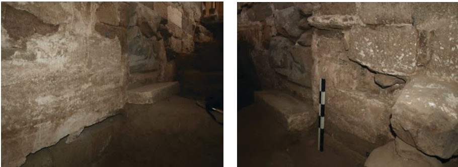
Figure 8: North face of the east minaret – left: step and original doorway blocked with stone (note the wood slot at the bottom of the wall plaster); right: the corner niche filled with stones of pillar foundations for the remodeled east riwāq.
