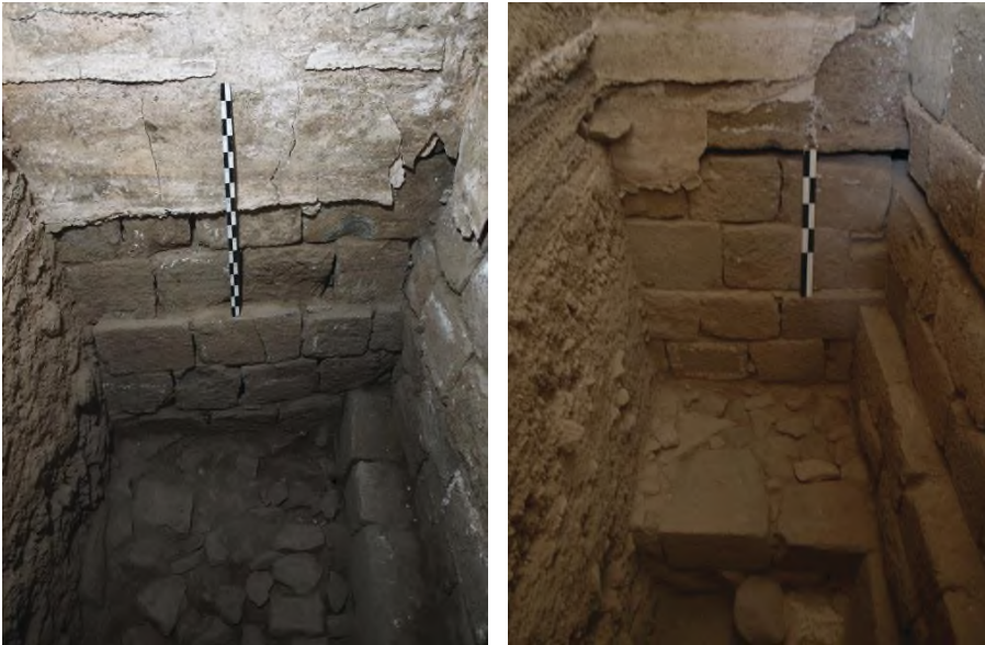
Figure 2: South interior corners of the mosque – left: southwest corner with minaret foundation in center, west wall foundation on right, and wall plaster continuous across the corner (the wood slot is at the top of the partially plastered course of facing blocks); right: the southeast corner after removal of wall plaster, the east wall foundation is in the center and the east minaret foundation is on the right, with the continuous wood slot visible in both foundations; note the bonding of stonework across both corners.
