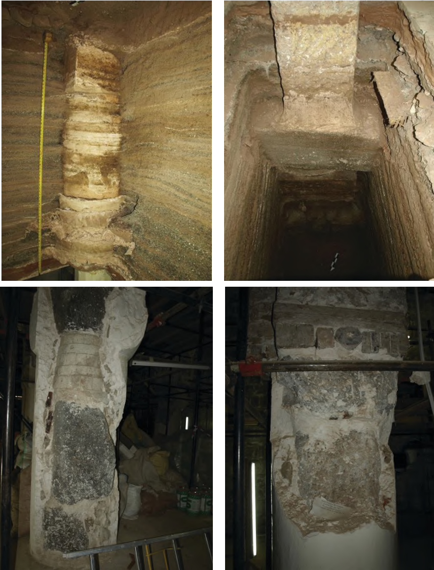
Figure 5: Pillars in the qiblah riwāq – upper left: original pillar below, a pre-Islamic pillar above; upper right: original pillar, base and foundation below, a later base and square pillar above; lower left: extant pillar of rough blocks and pre-Islamic spolia encased in plaster; lower right: composite stone and plaster pillar with wood beams.
