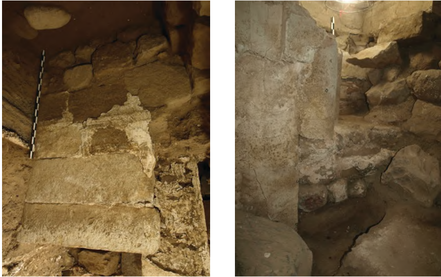
Figure 3: Central door in north (qiblah) wall – left: exterior porch structure from the north; right: engaged pillars of the initial mihrāb set on a bed of stones within the original doorway, the sill of which is visible at the bottom of the photograph.
