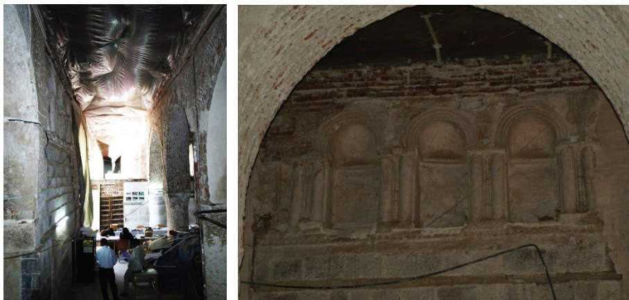
Figure 10: East face of the east minaret – left: view from from the south (arcading of the present east riwāq is visible at the left side of the photograph); right: arched niches in the east face of the east minaret, seen through present east riwāq arcading (note the truncated arched niche at the right side of the frieze).
