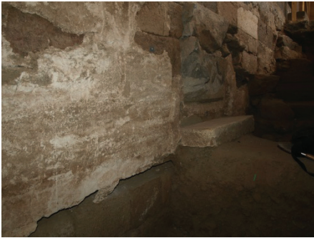
Figure 8: North face of the east minaret – left: step and original doorway blocked with stone (note the wood slot at the bottom of the wall plaster); right: the corner niche filled with stones of pillar foundations for the remodeled east riwāq.
