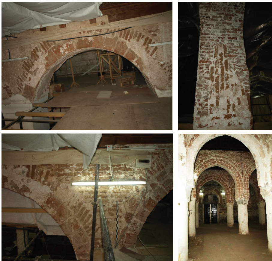
Figure 6: Arcading in the north riwāq – upper left: intact vertical brick lower course and radial brick upper course; upper right: rebuilt arch enclosing remains of the earlier vertical brick soffit; lower left: intact arch to left, rebuilt arch (transition to the present east riwāq) to right; lower right: arcading of the present east riwāq viewed from the north riwāq.
