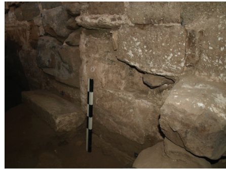
Figure 8: North face of the east minaret – left: step and original doorway blocked with stone (note the wood slot at the bottom of the wall plaster); right: the corner niche filled with stones of pillar foundations for the remodeled east riwāq.
