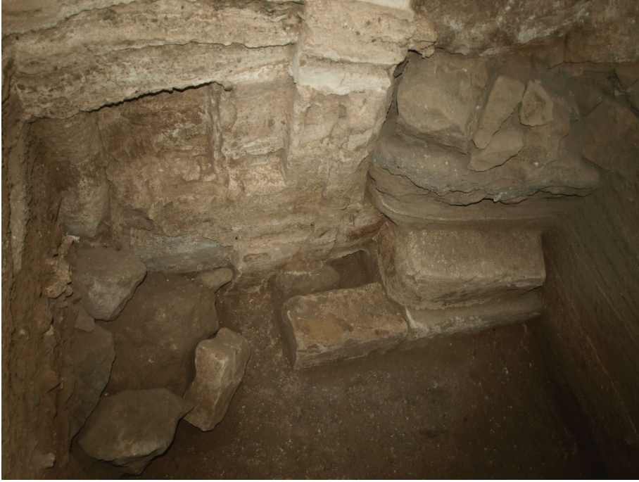
Figure 7: Original doorway (blocked with stones) and corner niche in the north face of the west minaret (the pillar visible on the left was inserted onto the corner niche to support arcading of the Yuʿfirid west riwāq).
