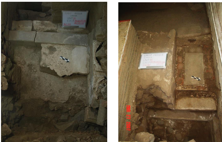
Figure 4: Doorways in the east wall – left: doorway into the 5th aisle of the north riwāq, from the east; right: doorway at the northeast corner of the north riwāq.
