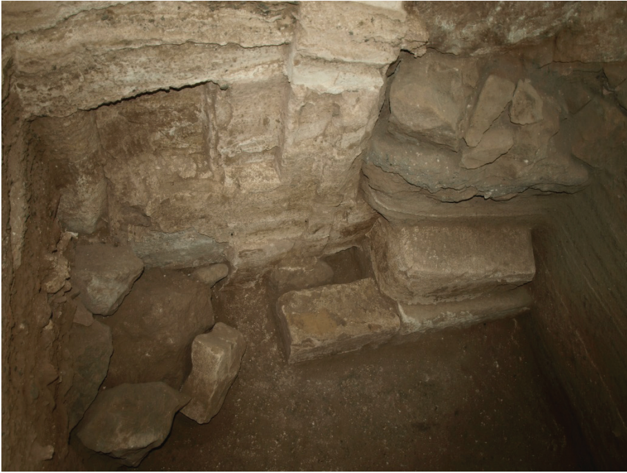
Figure 7: Original doorway (blocked with stones) and corner niche in the north face of the west minaret (the pillar visible on the left was inserted onto the corner niche to support arcading of the Yu‘firid west riwāq).
