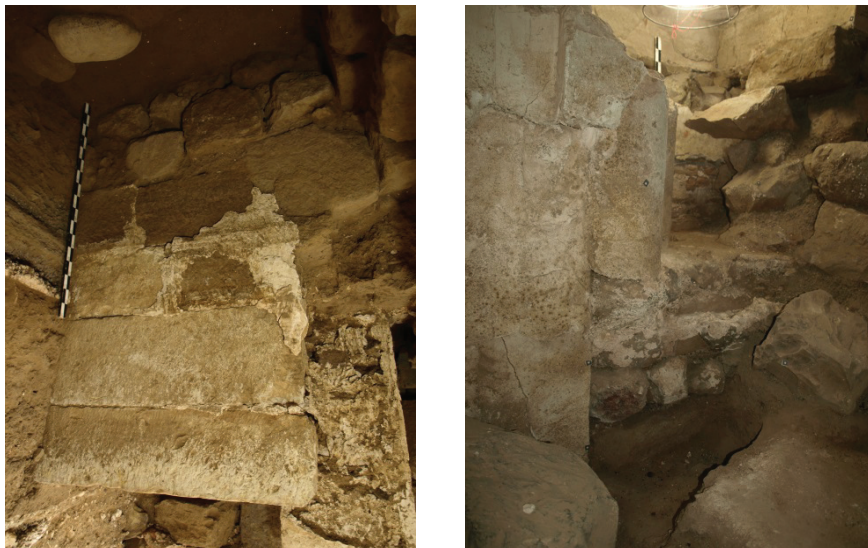
Figure 3: Central door in north (qiblah) wall – left: exterior porch structure from the north; right: engaged pillars of the initial mihrāb set on a bed of stones within the original doorway, the sill of which is visible at the bottom of the photograph.
