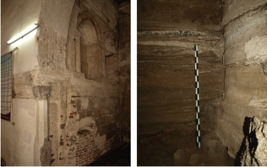
Figure 9: Northeast corner of the west minaret – left: pre-Islamic spolia supporting west riwāq arcading set against the east face of the minaret, with upper portions of the (original?) engaged pillar exposed to the left (the pair of arched niches and blocked doorway in the north face of the minaret are to the right); right: bottom of the engaged pillar set onto the south wall.
