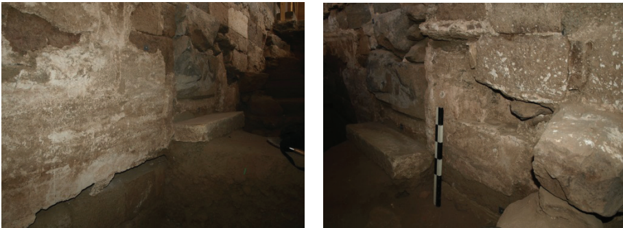
Figure 8: North face of the east minaret – left: step and original doorway blocked with stone (note the wood slot at the bottom of the wall plaster); right: the corner niche filled with stones of pillar foundations for the remodeled east riwāq.
